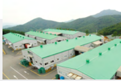
Deoksan Factory Click LVT, cutting & finishing
